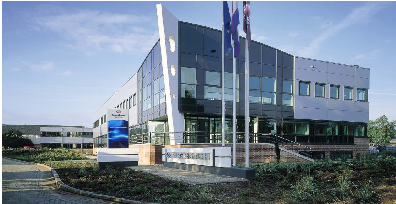
BRONKHORST HIGH-TECH HEADQUARTERS, THE NETHERLANDS
